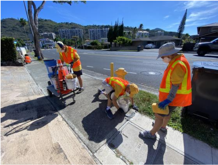
HK Lions filling in sidewalk cracks.
